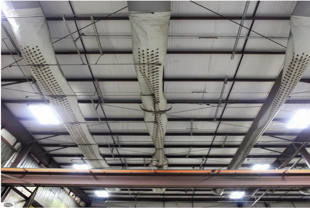
Overhead view of air recovery system
